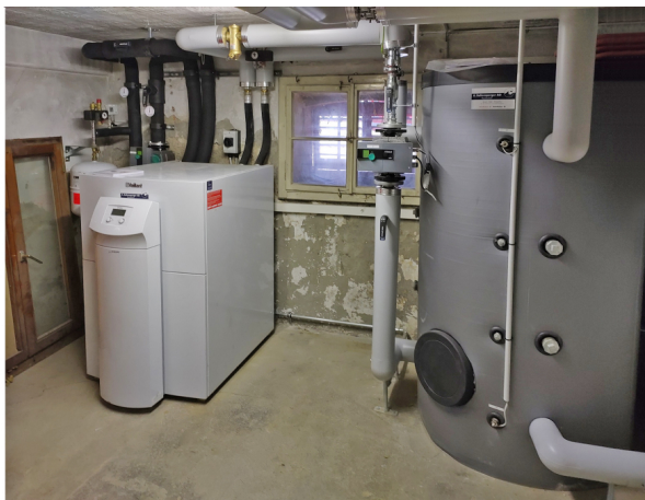
New geothermal heat pump replaces gas boiler in old building
