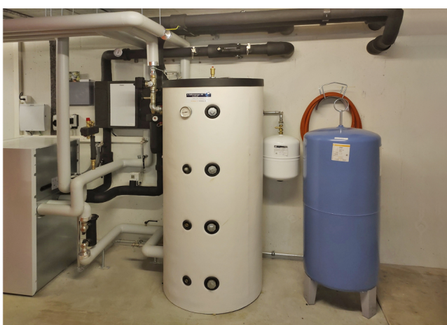
New geothermal heat pump in new building
