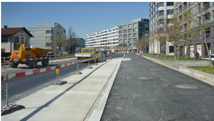
Bus stop with curbside slot drainage: ACO drainage slot in stainless steel
