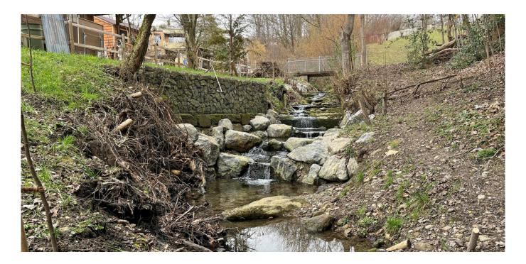
We developed the "Action plan for the implementation of measures addressing natural hazards" for the municipality of Männedorf. This included restoring the continuity of the village creek, with incrementally removing a dam while monitoring the effects. We assisted the municipality with hydraulic engineering and design measures to create a long-term stable and near-natural stretch of water.
